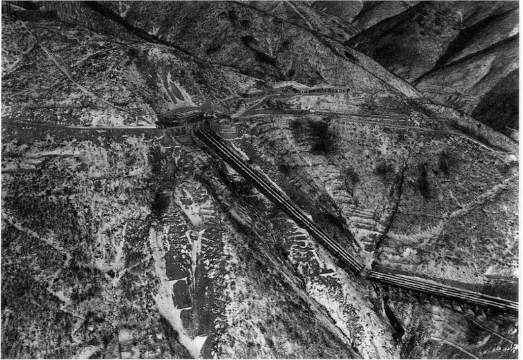
SITE OF THE DESTROYED BRIDGE SOUTH OF KOT'O-RI
