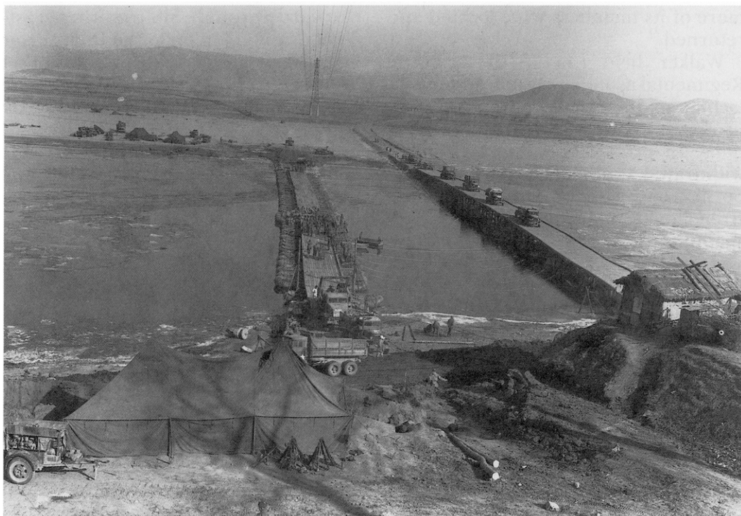
ALL BRIDGES OVER THE TAEDONG RIVER AT P'YONGYANG WERE DESTROYED after the Eighth Army withdrew south of the city.
